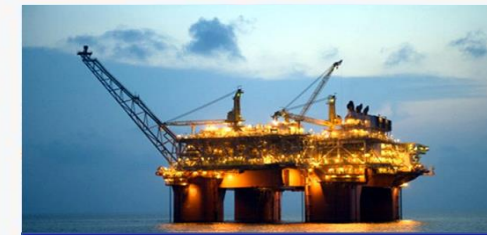
OFFSHORE PRODUCTION FACILITIES
